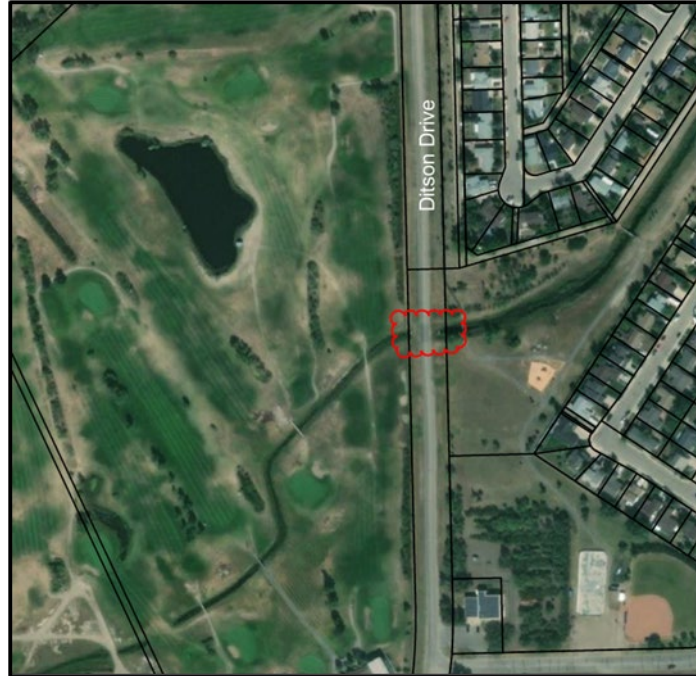
Figure 7.6: Ditson Drive Culvert Failure
