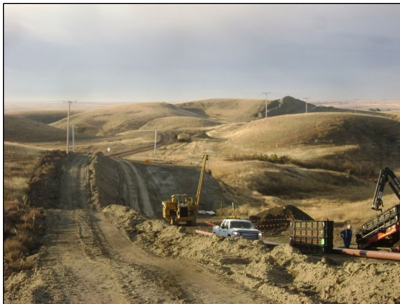
Figure 3.3: Installation of Raw Water Supply Pipeline (2011)
