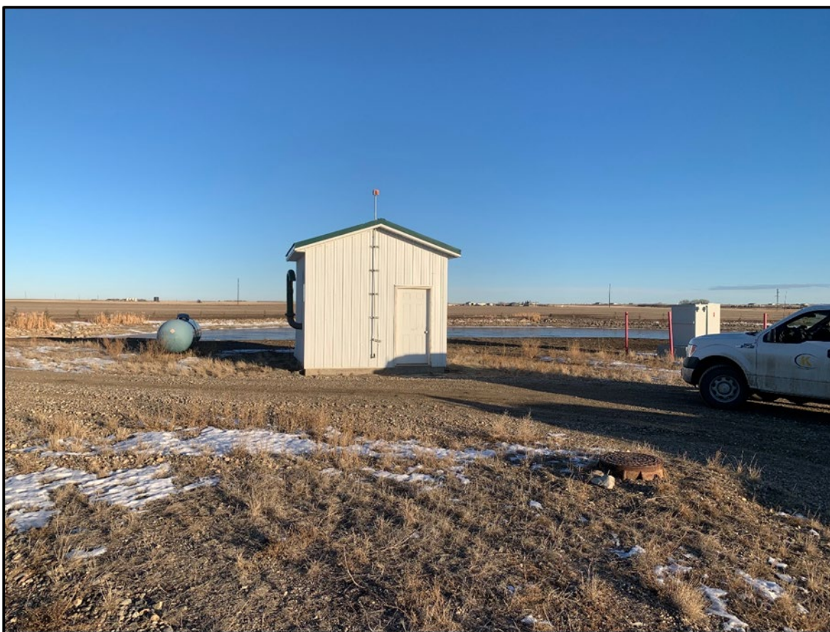
Figure 5.4: Industrial Lift Station
