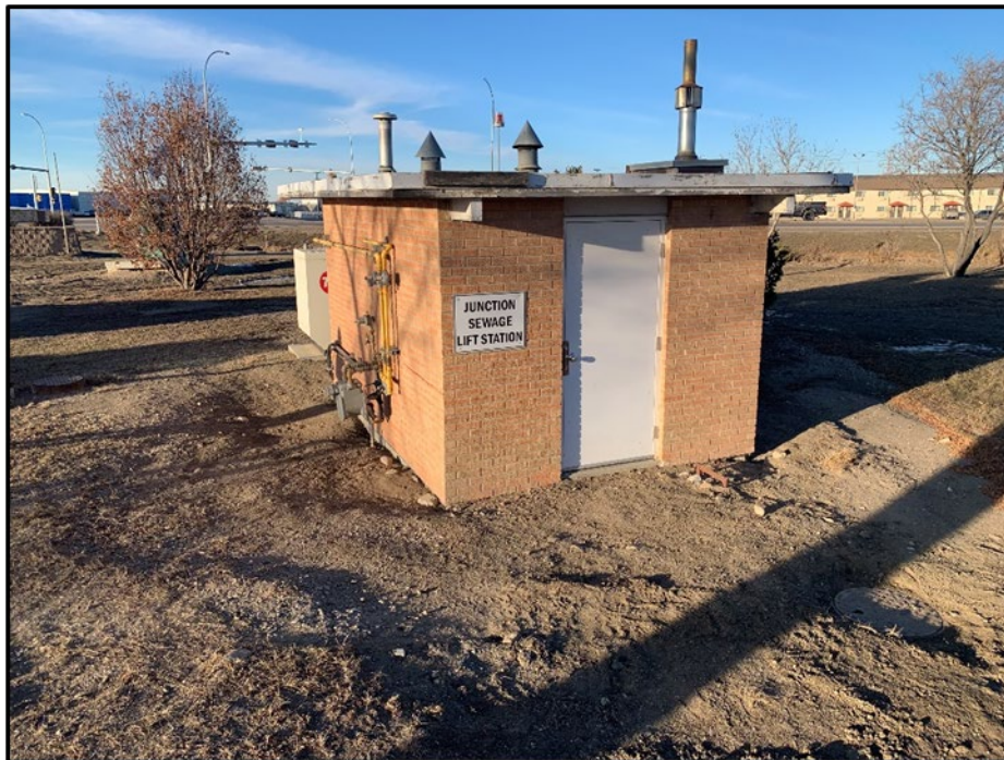
Figure 5.2: Highway 7 & 21 Lift Station
