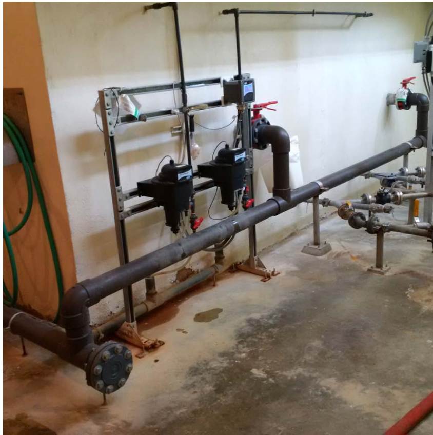
WTP – Turbidimeters
