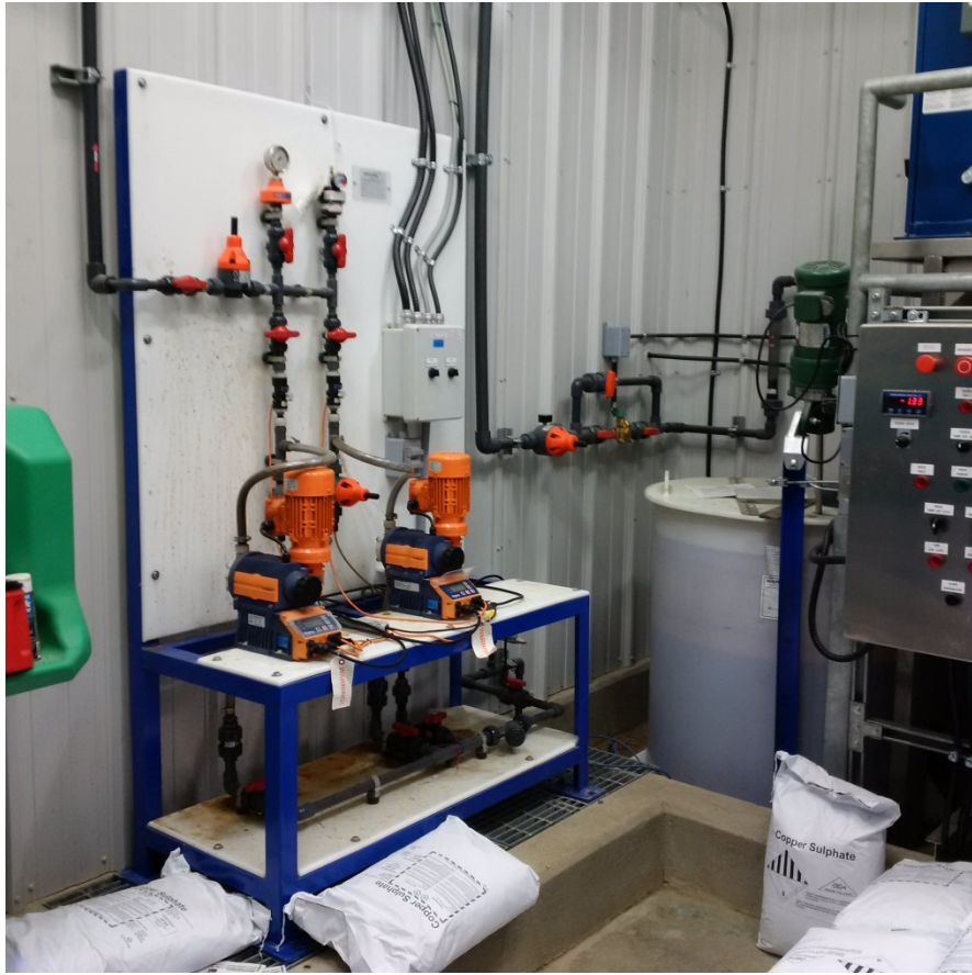
CN Pumping Station – Potassium Permagnate System
