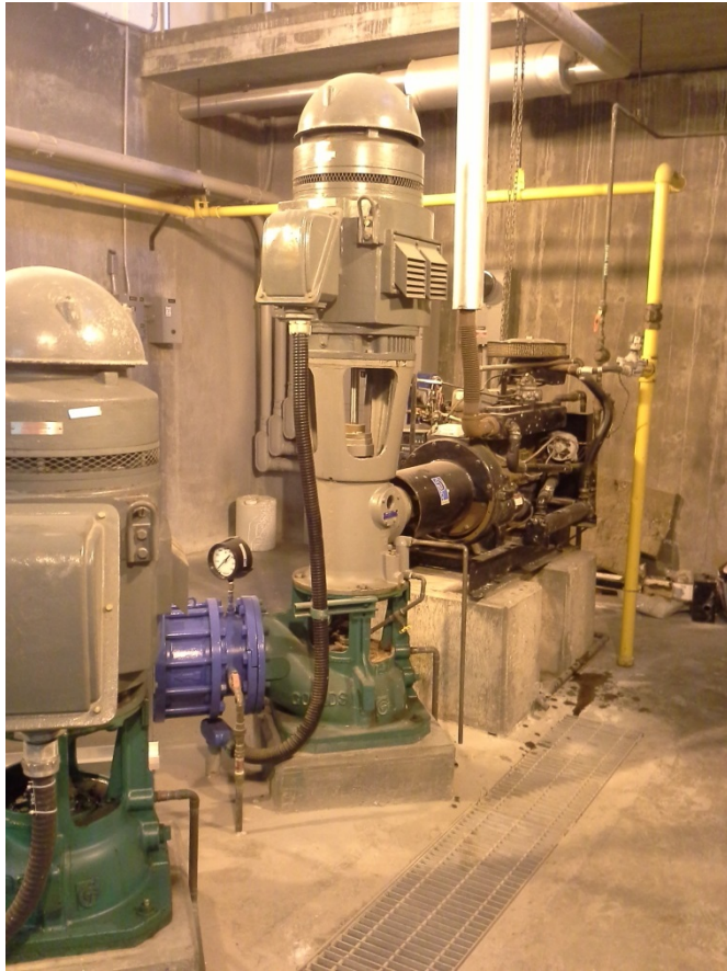
WTP - Engine Driven Pump
