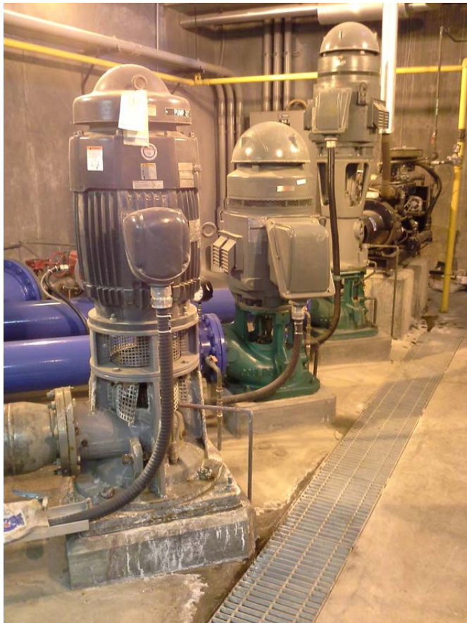
WTP – High lift distribution pump
