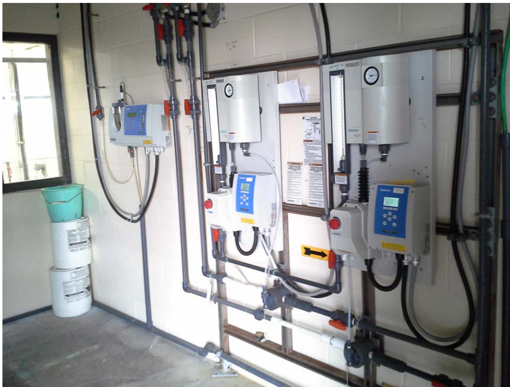
WTP – Gas Chlorination System
